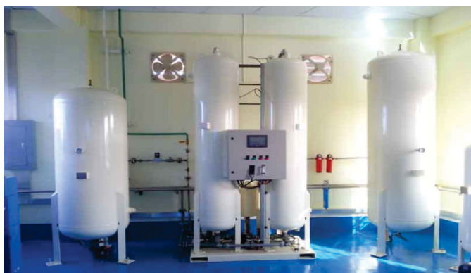
Oxygen Generator for 4 to 20 Cylinder. per day
